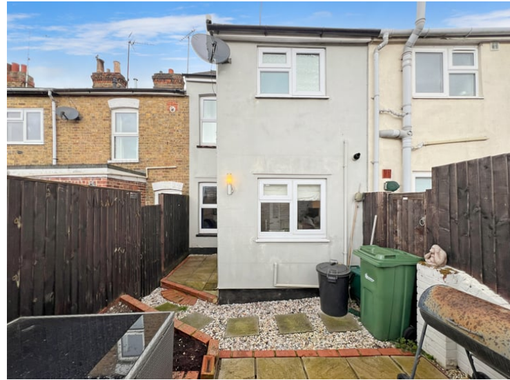
Courtyard garden low maintenance design.
