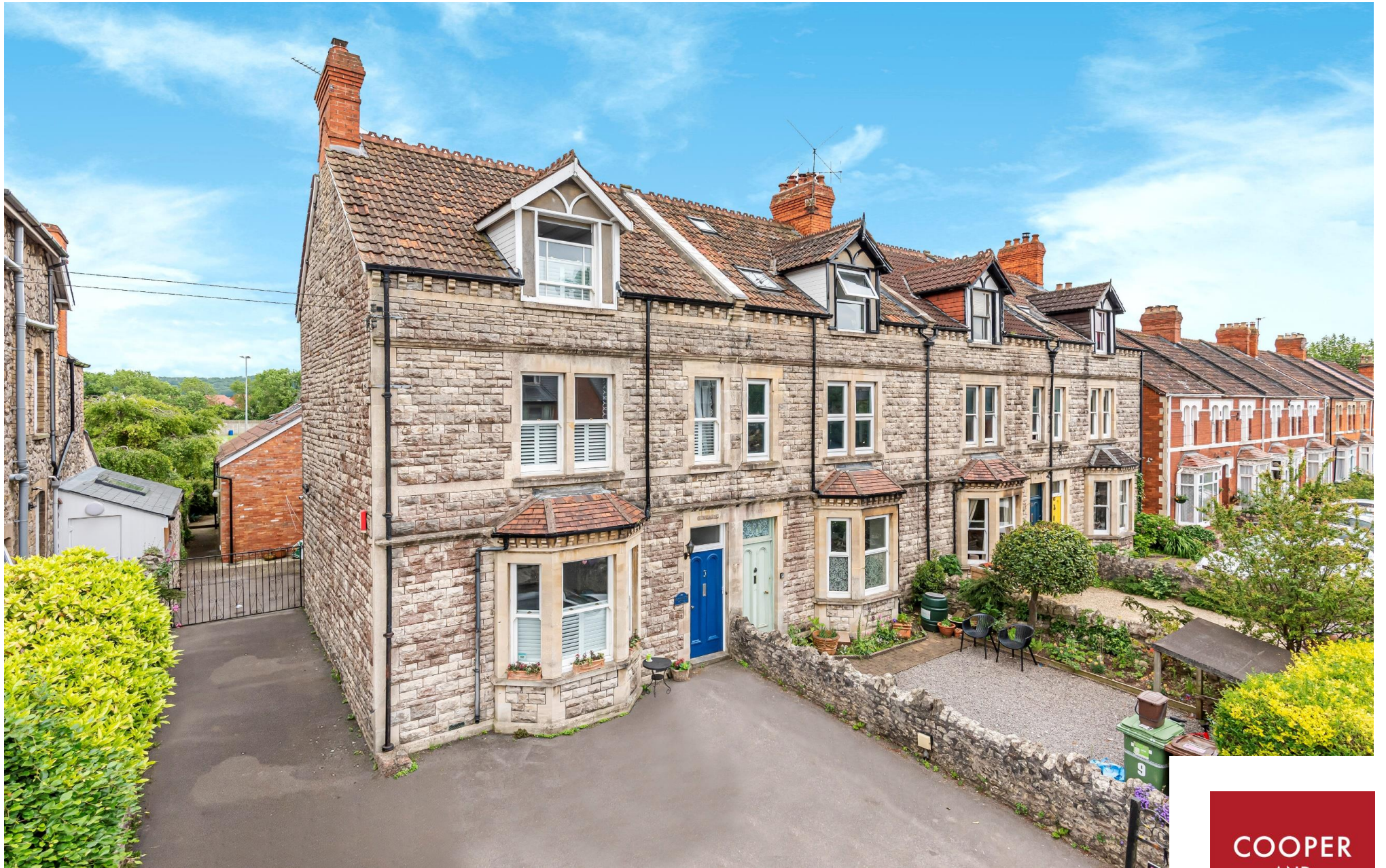
Glengarth House, Glastonbury Road, Wells, BA5 1TW
