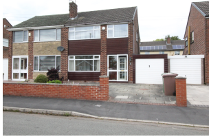
Porch with PVC sliding Patio doors.
