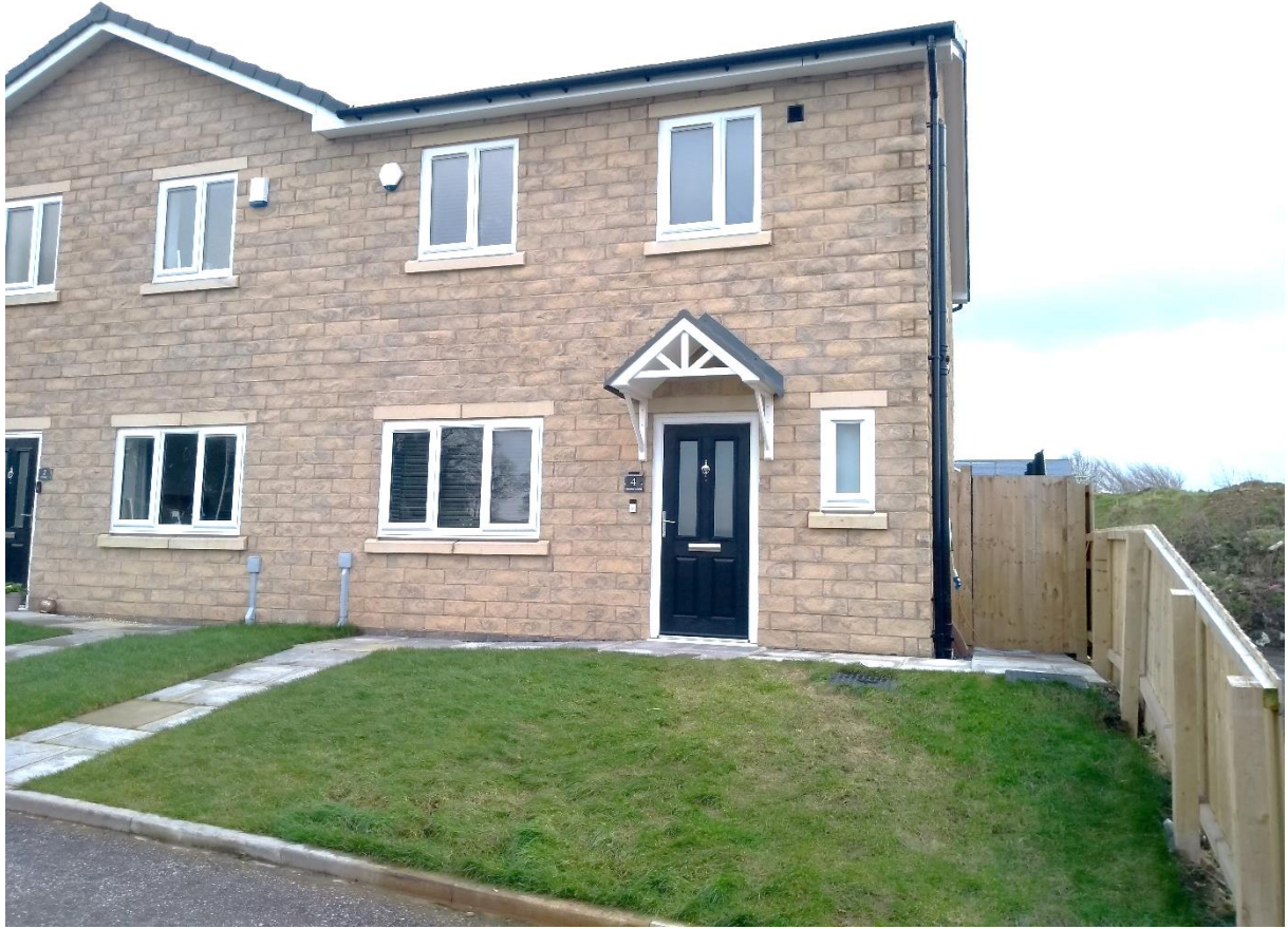
Westerly view from the front of the property.
