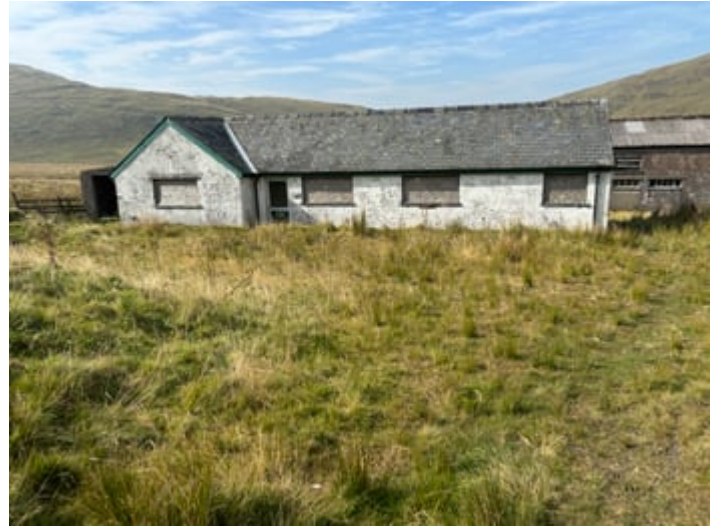
SETTING FROM THE SOUTH APPROACH
