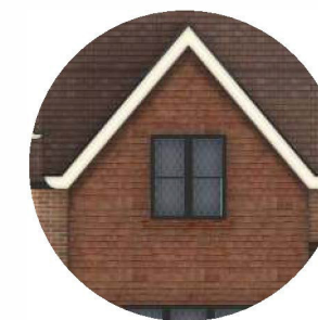
Principal gable details with vertically hung tiles.
