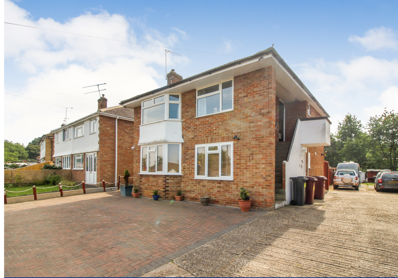
Amblecote Road, Tilehurst, Reading.
