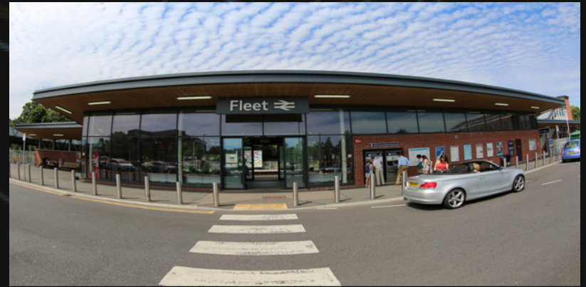
Fleet Mainline Railway Station
