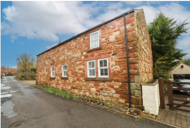
EXTERNAL FROM ROADSIDE
