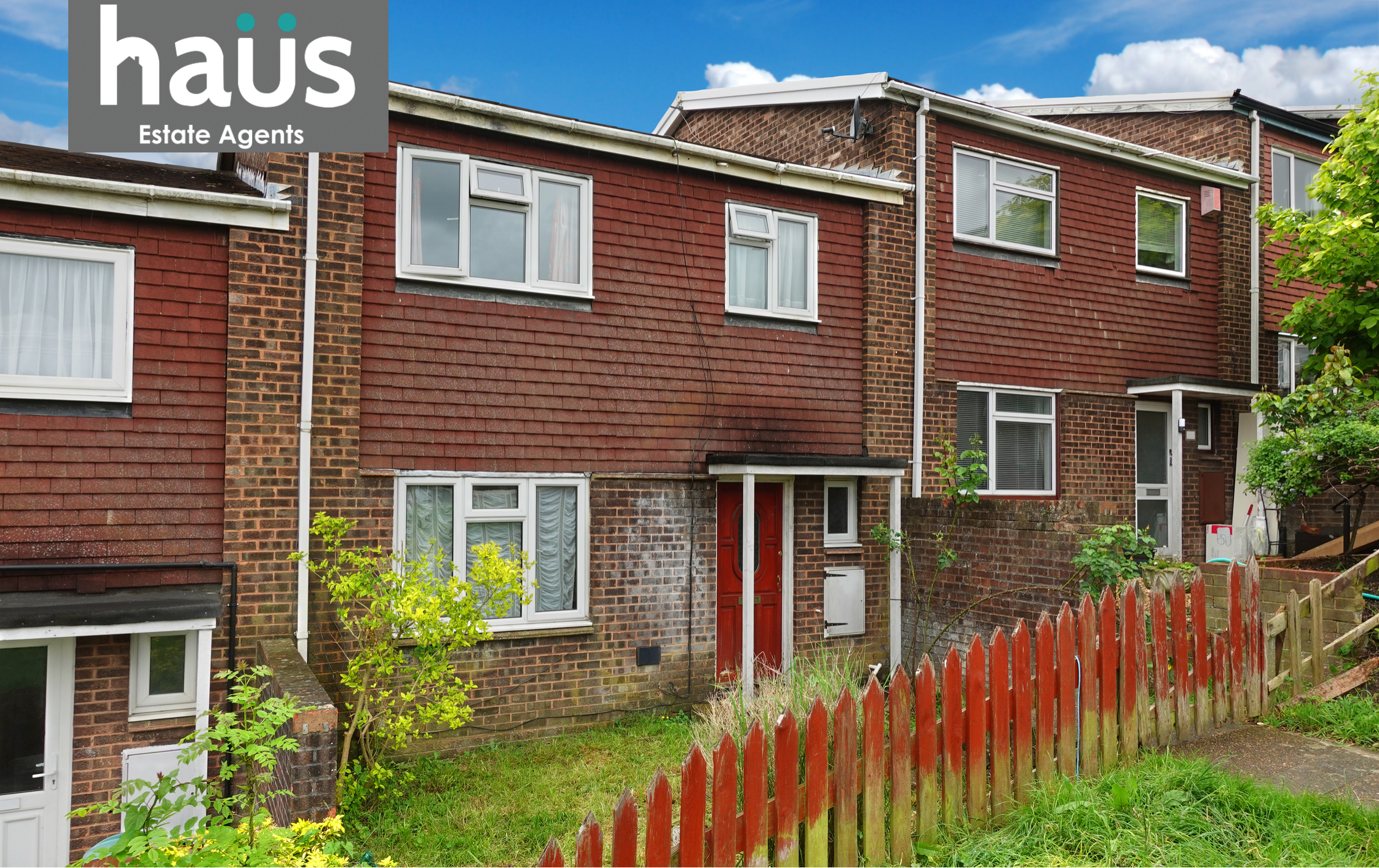
Three Bedroom Terraced House Charter Street, Chatham, Kent, ME4 5RJ
