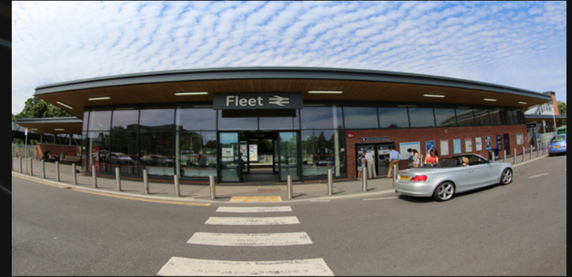
Fleet Mainline Railway Station
