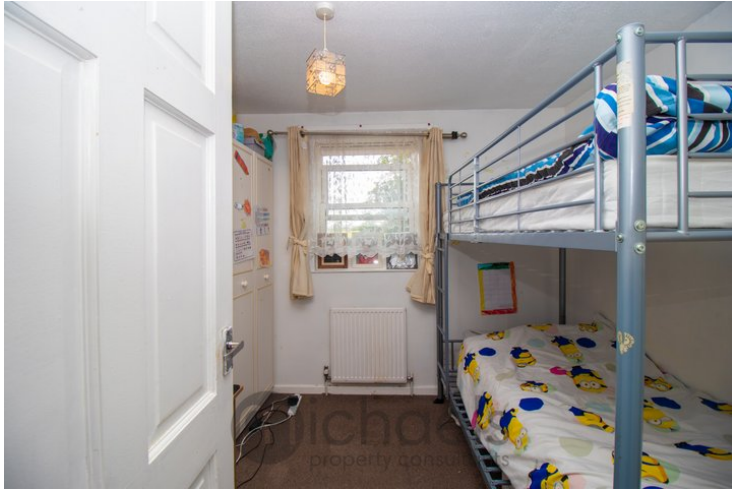
UPVC window to rear, radiator
