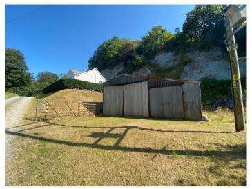
24' 0" x 28' 0" (7.32m x 8.53m) A steel and zinc cladding construction, concrete base with inspection pit, double doors to front. Please note there is potential of a electrical connection immediately adjoining the Workshop (STC).
