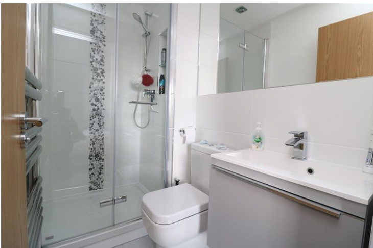
Shower cubical, close couple WC, wall hung vanity wash hand basin, heated towel rad, extractor fan, tiled splashbacks, spotlights.
