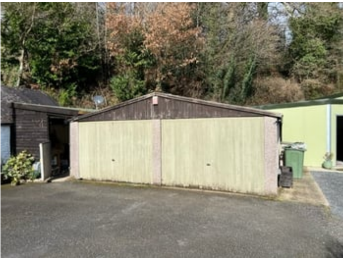
Covered Tractor/Log/Store Processing Building.
