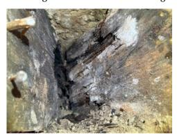
Decay to bressummer beam end and joist end above bay window area to ground floor room front
