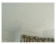
Penetrating dampness to ceiling fabric to 1st floor room front left
