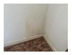
Mould growth due to condensation to 1st floor room rear left
