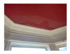
Penetrating dampness to ceiling, cornice and wall fabric to ground floor room front
