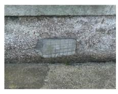
Blocked sub-floor vent to rear elevation
