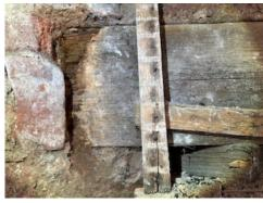
Decay to timber lintels above front door
