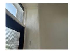
Penetrating dampness to wall fabric to ground floor vestibule
