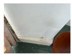
Penetrating dampness to wall fabric to 1st floor room front left
