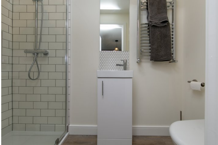
Shower cubical, vanity wash hand basin, close coupled WC, heated towel rail.
