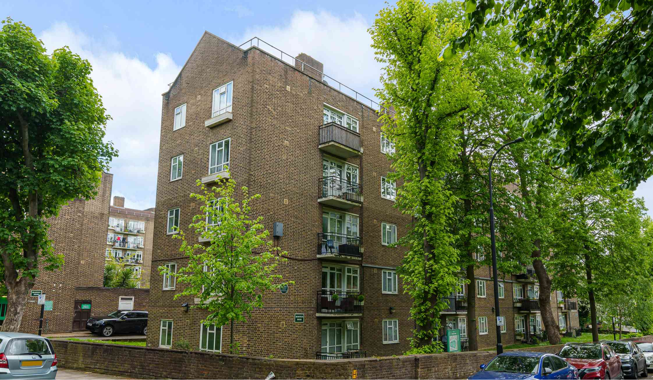
Mortimer Crescent, London, NW6 5UT
