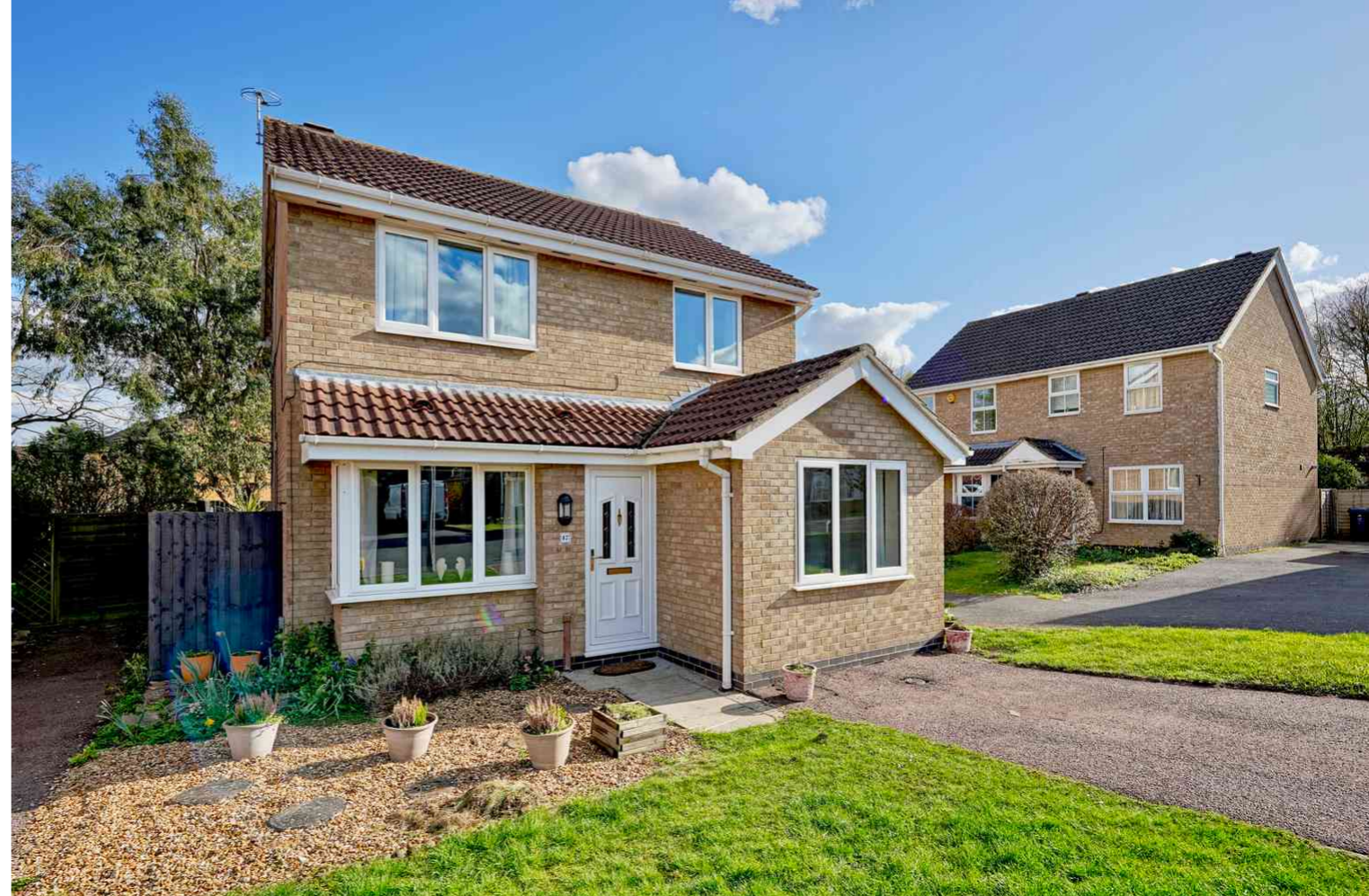
Ennerdale Close, Stukeley Meadows PE29 6UU
