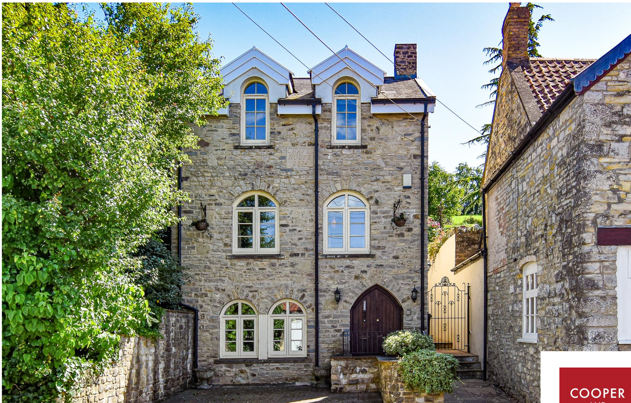
Chapel House, Coombe Batch, Wedmore BS28 4DU
