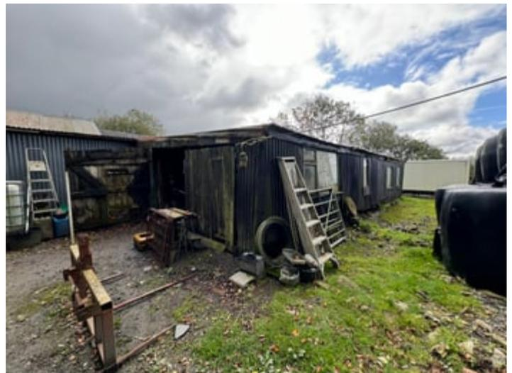
24' 0" x 18' 0" (7.32m x 5.49m) of timber construction with zinc cladding with vehicle inspection pit, side windows, concrete base, multiple sockets, connecting door through to:
