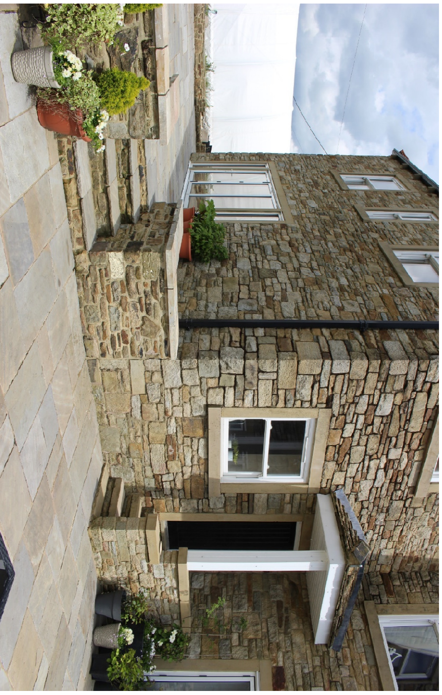
Rear Utility Entrance
