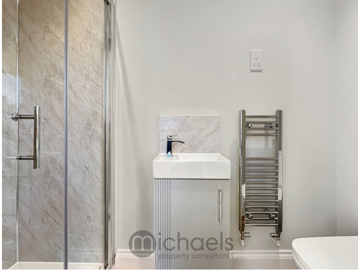
W.C., shower cubicle, vanity wash hand basin, radiator
