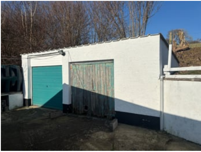
DETACHED DOUBLE GARAGE/WORKSHOP (SECOND IMAGE)
