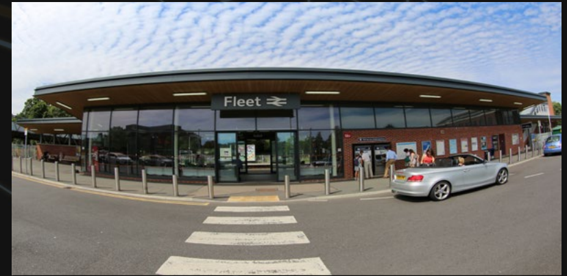
Fleet Mainline Railway Station
