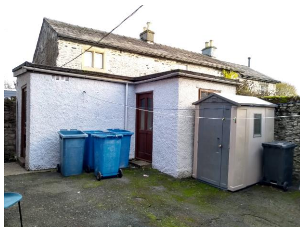
Detached Cold Room:
