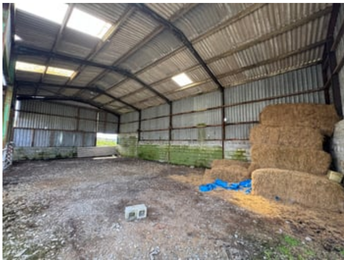
60' 0" x 30' 0" (18.29m x 9.14m) of steel frame with box profile cladding and cement fibre roof.
