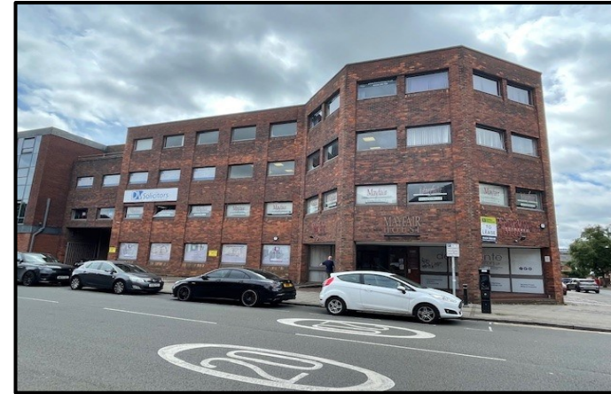
Existing Office Building
