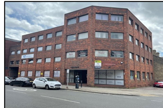
Existing Office Building
