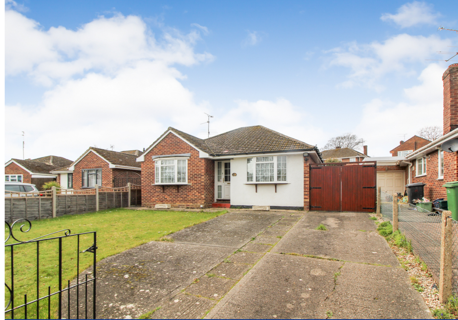
Kirkfell Close, Tilehurst, Reading.
