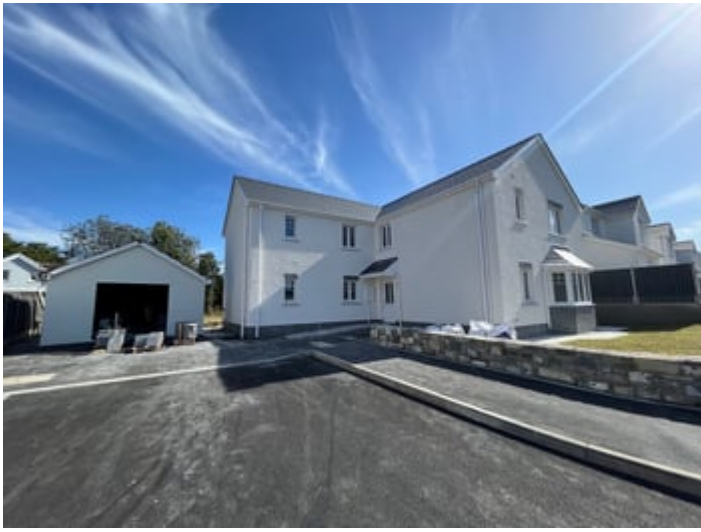
A stone walled forecourt with lawned area.
