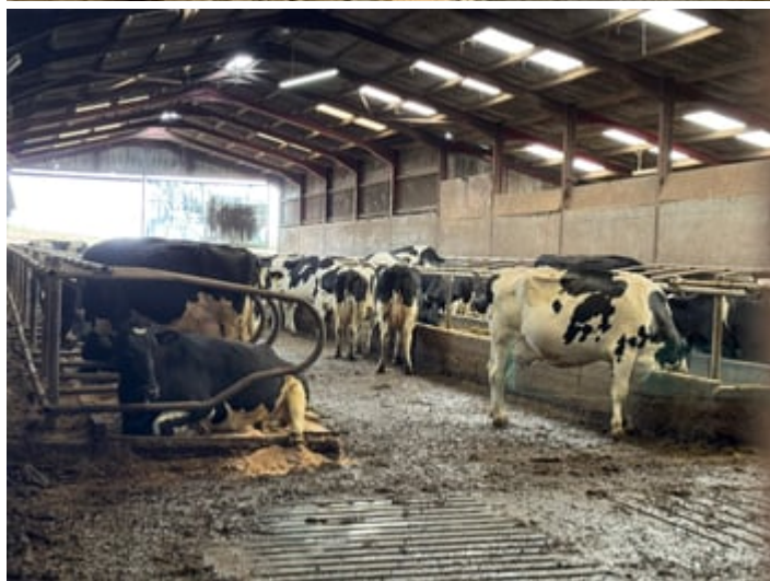
180' 0" x 45' 0" (54.86m x 13.72m) steel frame with cement fibre roof, concrete shuttered sides, 120 cubicles and slatted floor with slurry store.
