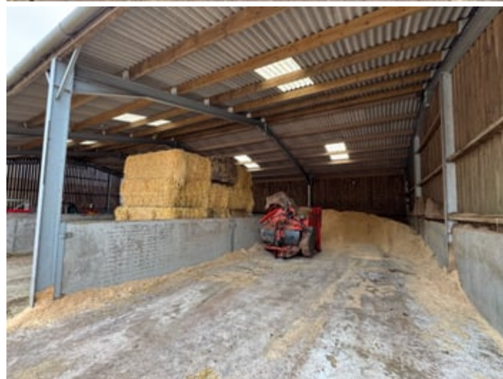
85' 4" x 45' 11" (26.01m x 14.00m) steel frame, Yorkshire boarding to sides, cement fibre roof, open onto concrete forecourt
