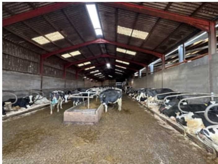
79' 9" x 46' 11" (24.31m x 14.30m) steel frame, box profile cladding, cement fibre roof, 40 cubicles and loose housing with central feed troughs.
