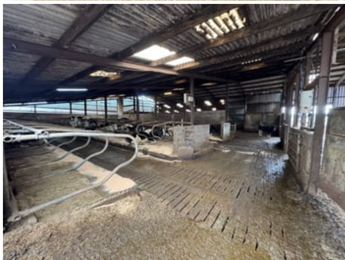
95' 0" x 75' 0" (28.96m x 22.86m) steel frame, cement fibre roof, slatted flooring with slurry store beneath, 60 cubicles.
