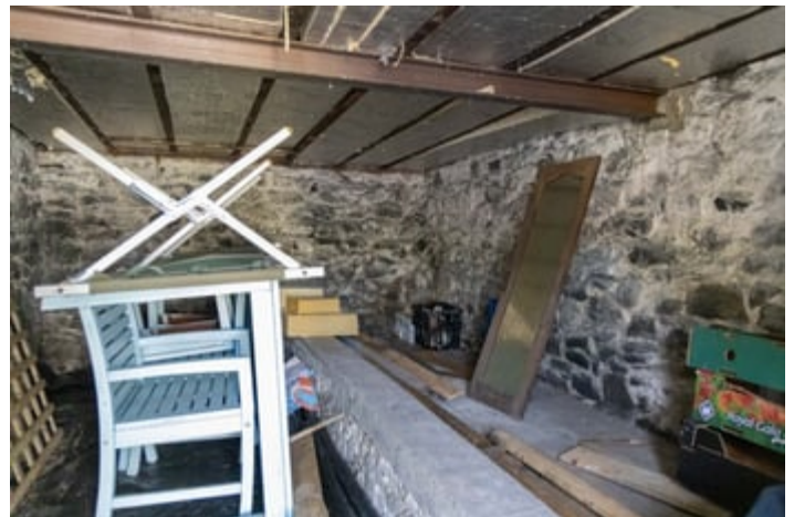
Accessed Externally from the front providing excellent additional storage space
