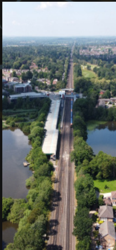
Rail Line/Fleet Pond
