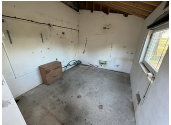
11' 9" x 9' 8" (3.58m x 2.95m). Recently re-roofed.
