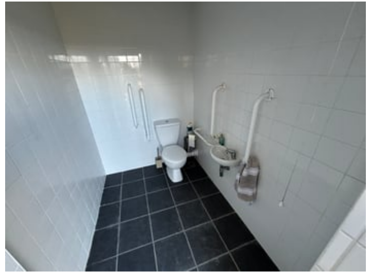
Being Disabled friendly with low level flush w.c., and wash hand basin.
