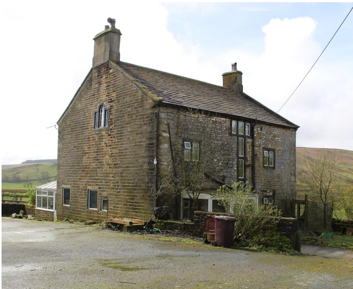
Harrop Lodge Farmhouse – Rear Elevation
