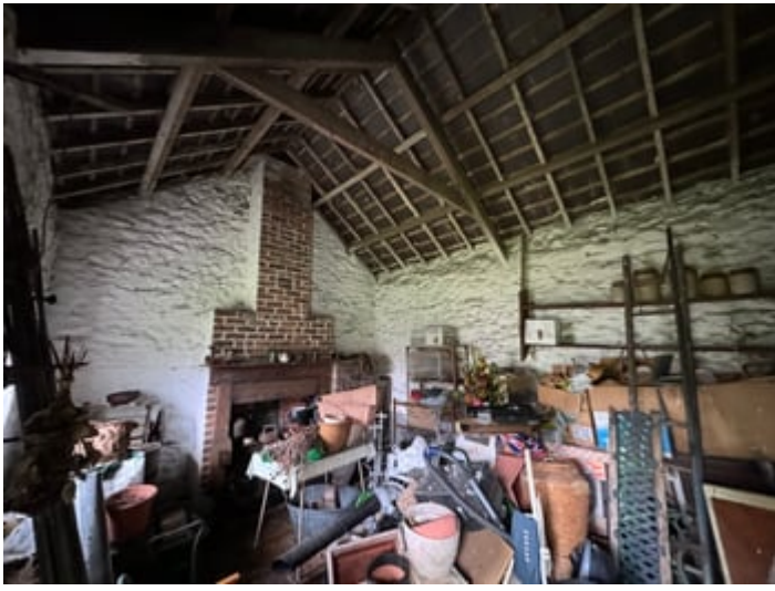
Timber Shed (14'2" x 8'3") with double timber doors to front, concrete base, side window.
