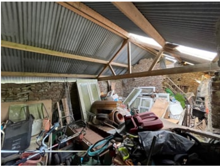
Wooden and Corrugated iron Open Sided Barn
