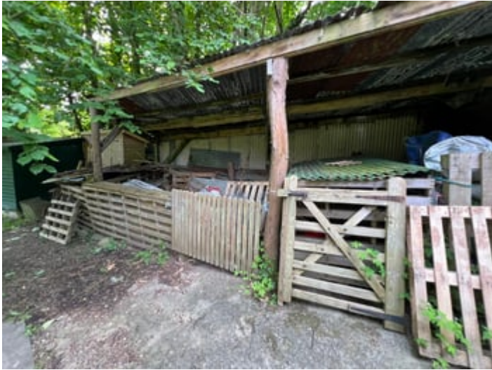
Of timber construction with zinc roof.
