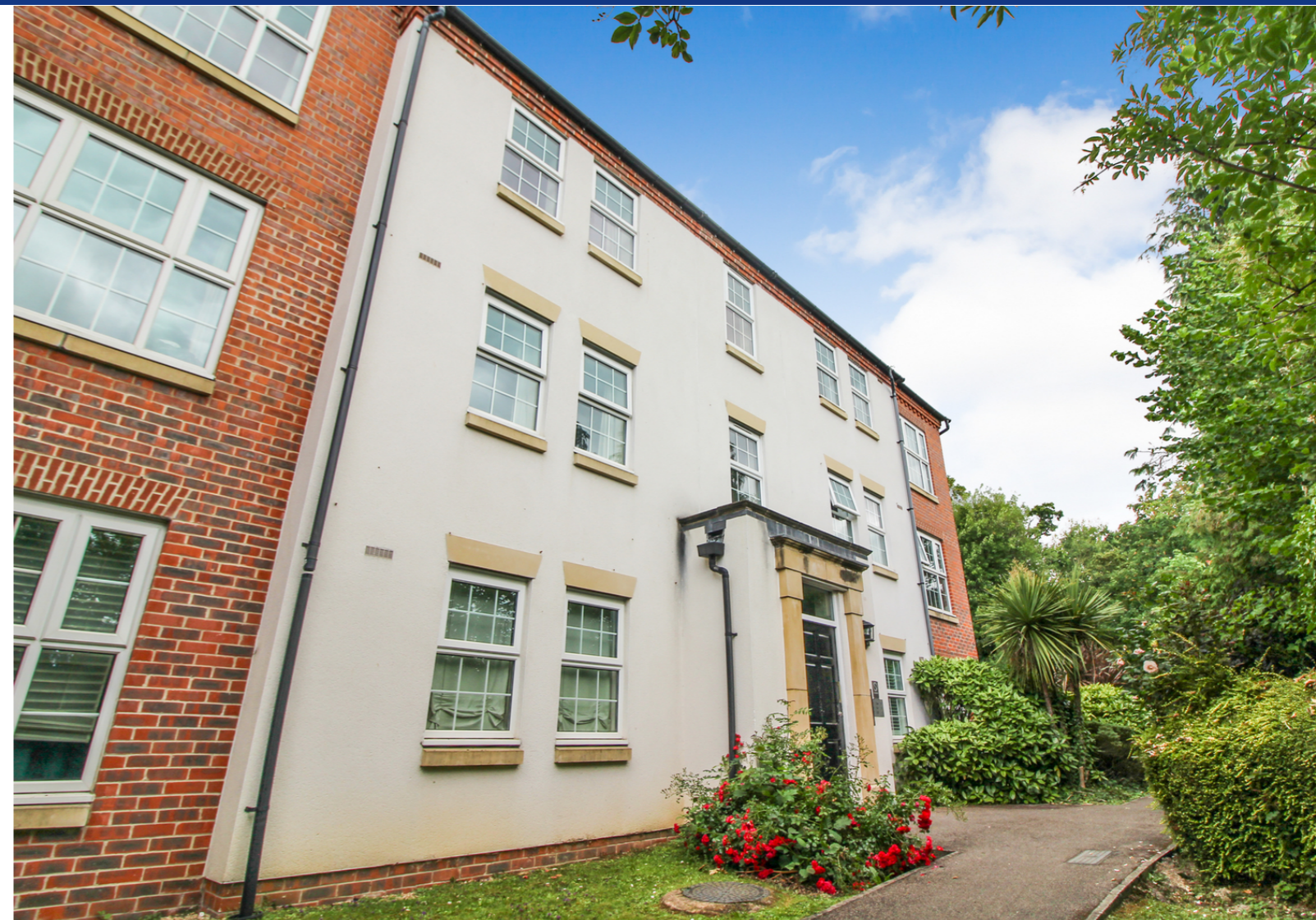
Lippincote Court, Oxford Road, Tilehurst, Reading.
